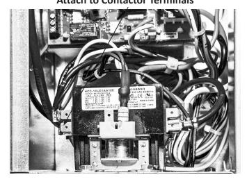
NOTE: Three phase models do not have open terminals on contactor. Remove two wires from contactor, install supplied electrical connector and connect wires.
