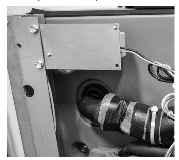
7. Route and secure line voltage wires (black & white) with the power cord. Wires must enter control box through line voltage Heyco fitting and attach to L1 and L2 contactor terminals.
