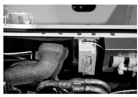
**Step 2** Route line voltage wires (black & white) through line voltage Heyco fitting. Disconnect L1 & N wires and install L1 & N of wiring adapter to the incoming power supply wires. Connect removed wires and LuminIce® wires to adapter.
