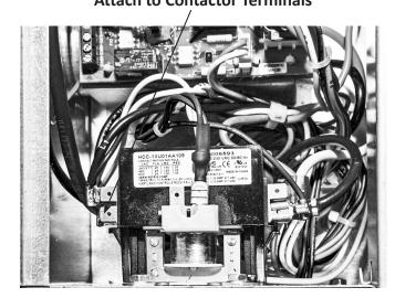
NOTE: QuietQube models do not have open terminals on contactor. Remove two wires from contactor, install supplied electrical connector and connect wires.
