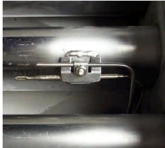
Typical high-limit/sensor probe locations and mounting hardware.
